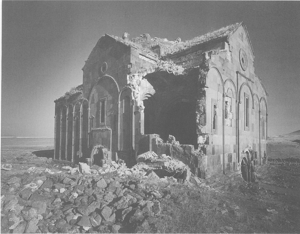
Figure 11 Ani Cathedral, view from the northwest
